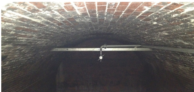
Storm Blaster installed in a covered tank
