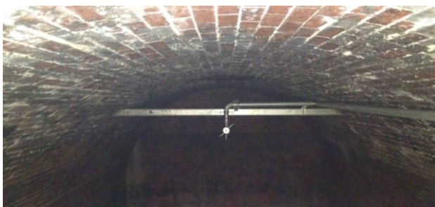
Storm Blaster installed in a covered tank
