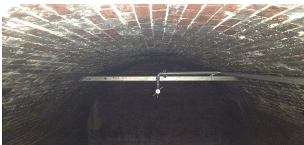
Storm Blaster installed in a covered tank
